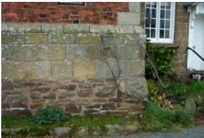
Plinth of the former Free School showing Enchmarsh stone below the more commonly used Hoar Edge grit-stone.
