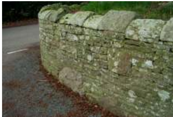
Stone wall with 'cock and hen' copings
